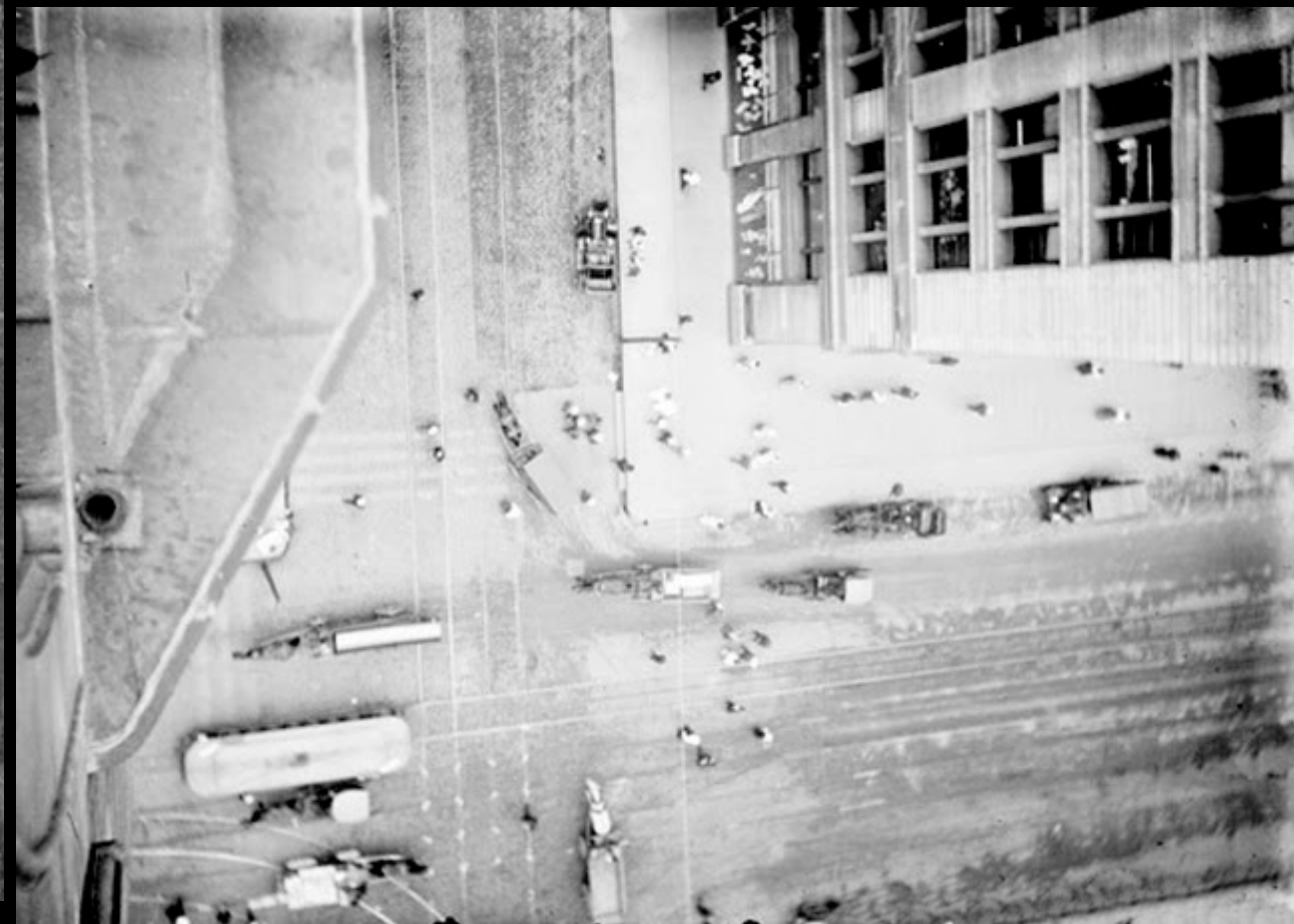
View of Randolph and State from the roof
