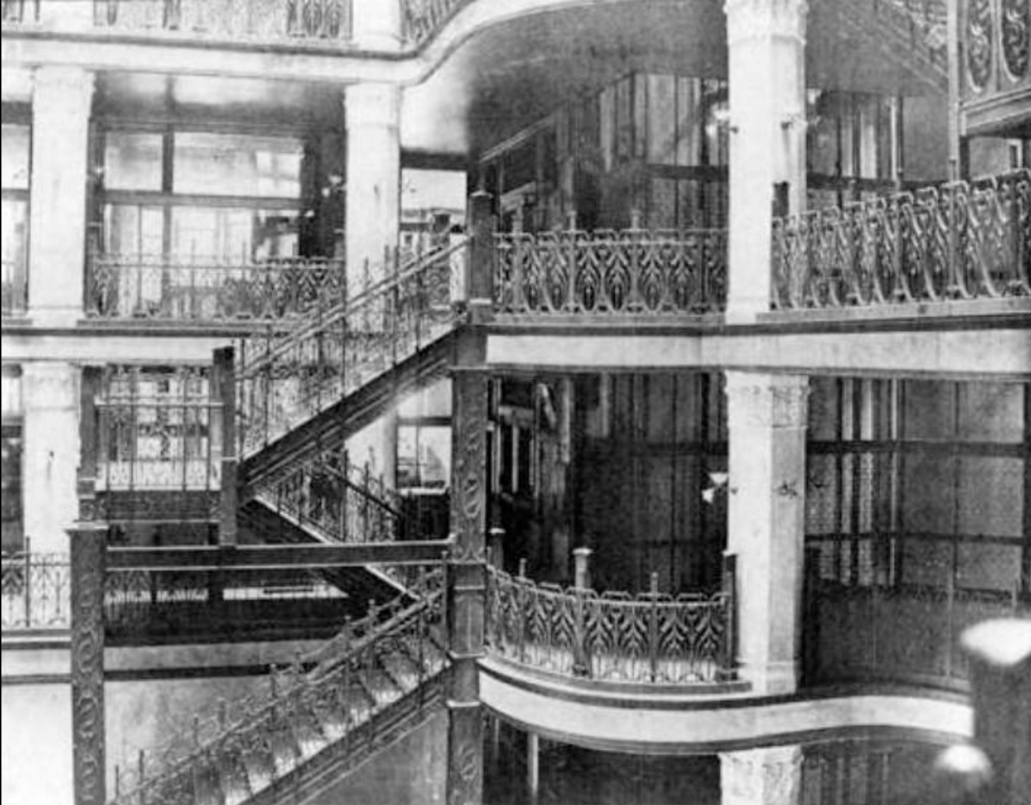
Stairways and Galleries of the Masonic Temple, 1892
