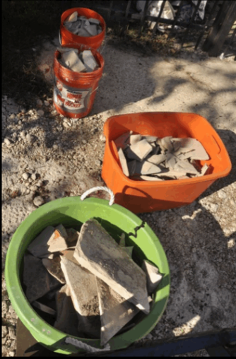
Reclaimed stones to be broken up and used within the rain garden
