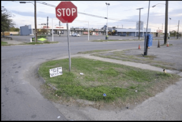
Unkempt parkway before work began
