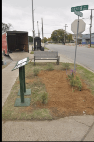
Completed curb, with native plants, covered in decomposed granite.
