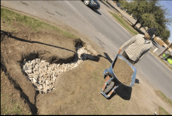
Laying the stones
